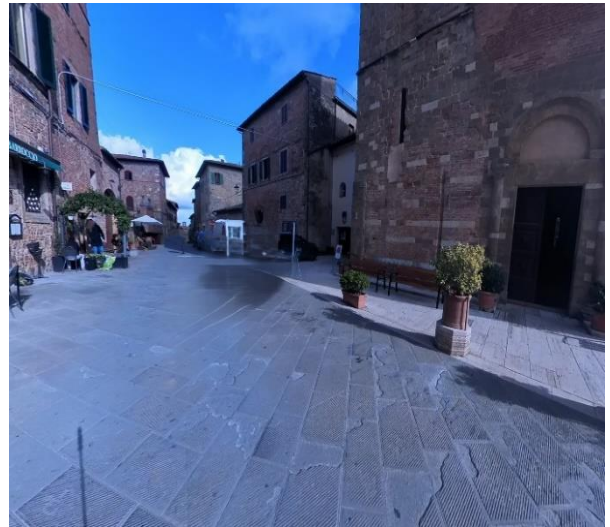
49 entrance portal on the main façade
