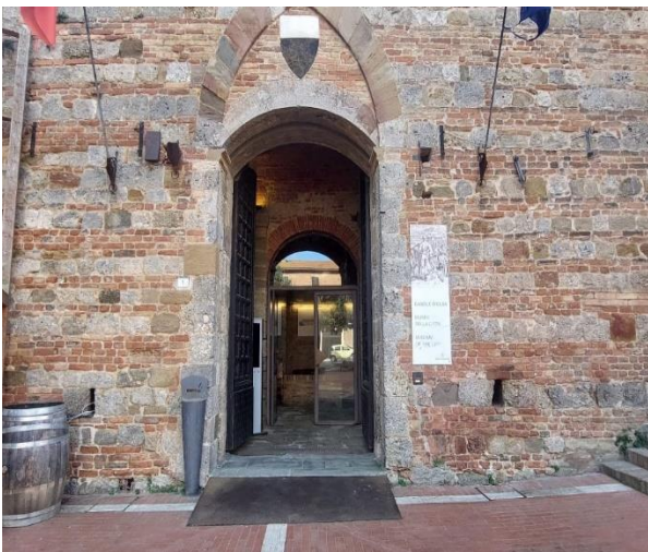
16 ramp entrance to the Town Hall
