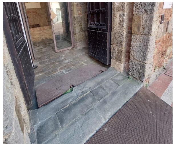
17 External and internal ramp
